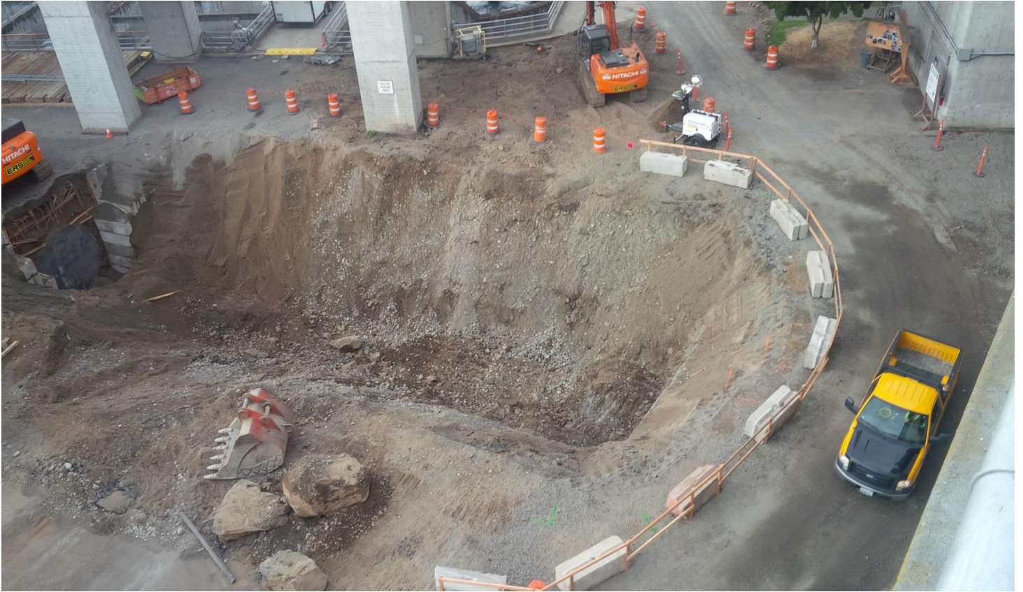
AWS digging resumes.
