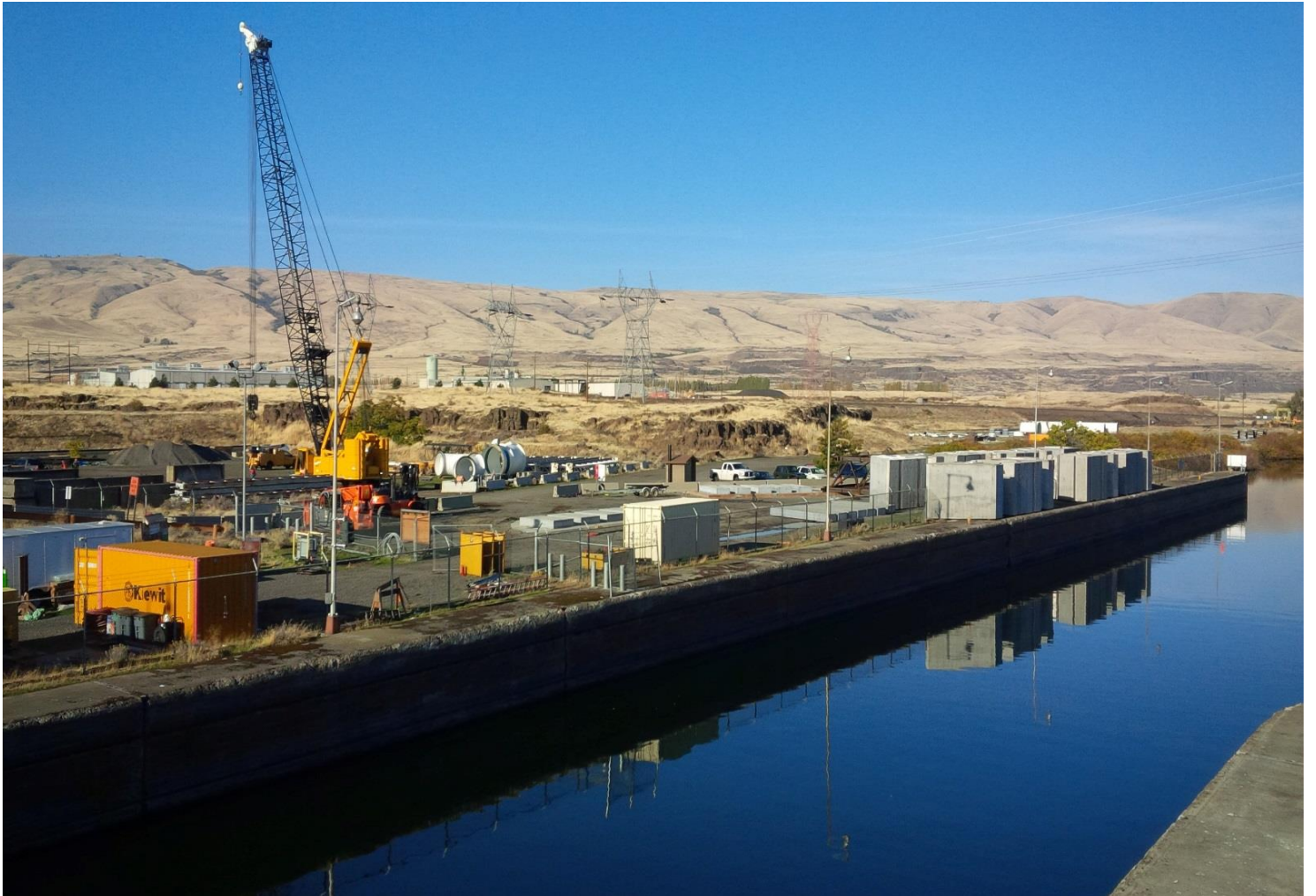
AWS pipes staged on WA shore ready for install
